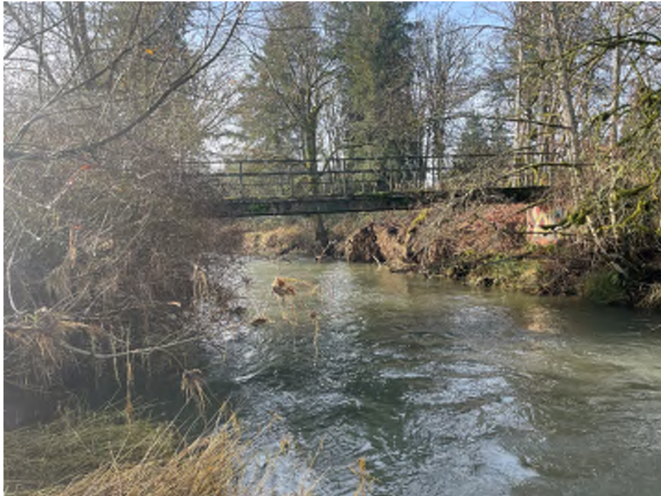
Photo 2 – Gordy Jolma No 5 Elevation view.
