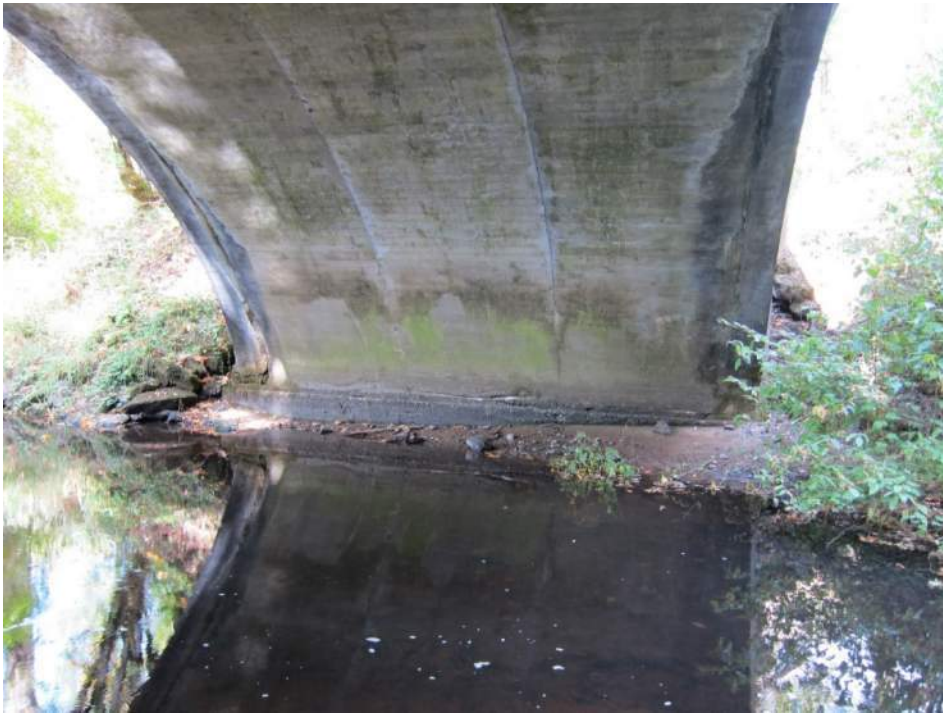
Photo 5: Salmon Creek Bridge – North Abutment
