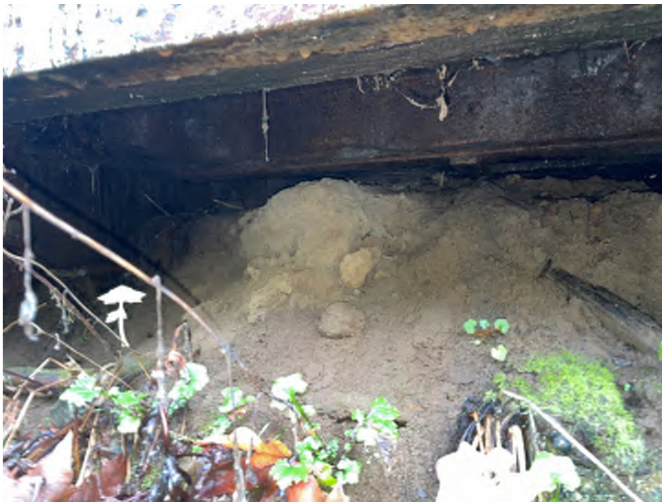
Photo 6 – Gordy Jolma No 11 Interior beam severe corrosion, pitting and loss of section.
