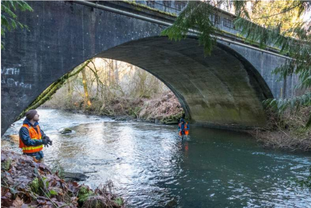
Photo 1: Salmon Creek Bridge – Looking downstream
