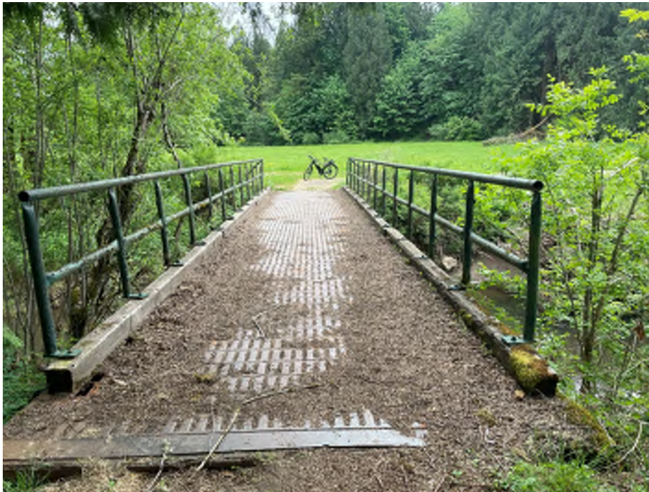
Photo 1 – Gordy Jolma No 8 Approach and Deck view.
