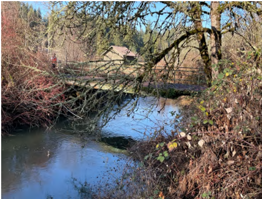
Photo 2 – Gordy Jolma No 3 Elevation view.
