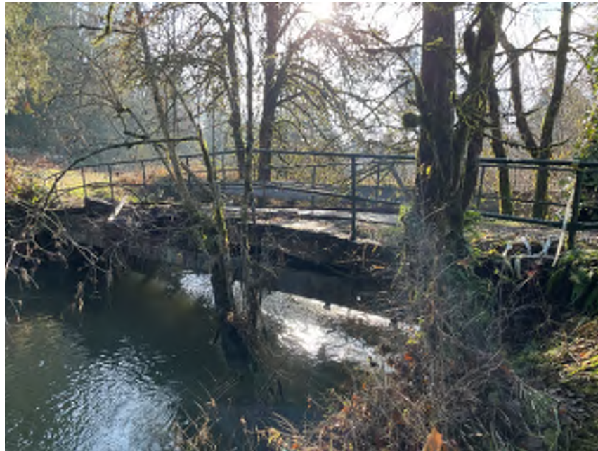
Photo 2 – Gordy Jolma No 4 Elevation view.
