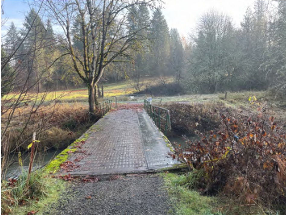
Photo 1 – Gordy Jolma No 1 Approach and Deck view.
