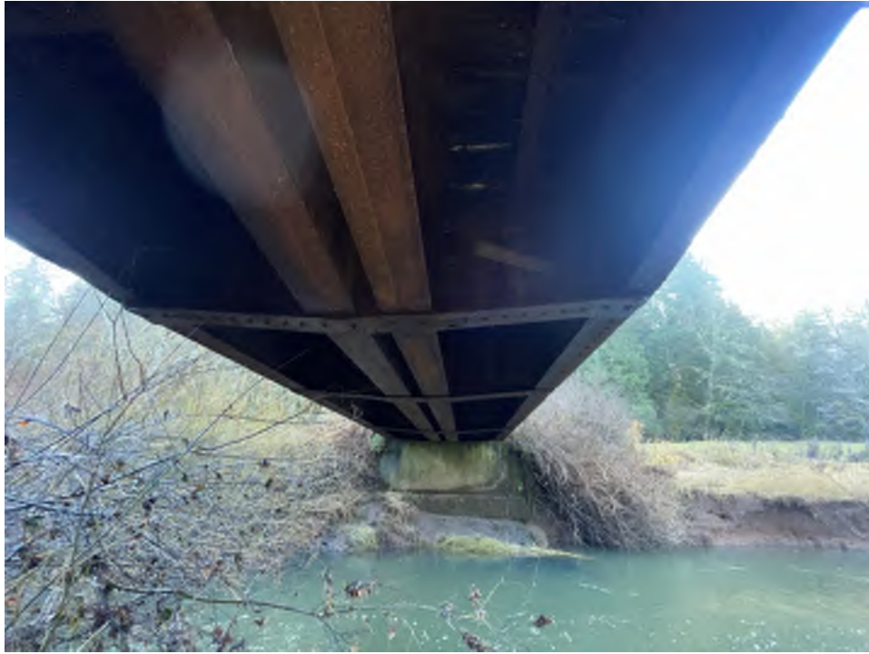
Photo 3 – Gordy Jolma No 9 Abutment and Railcar underside
