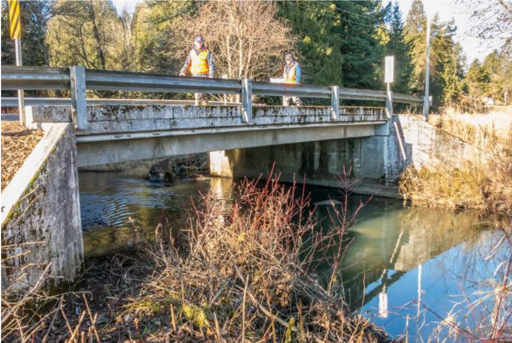
Photo 1: Smith Bridge – Looking downstream
