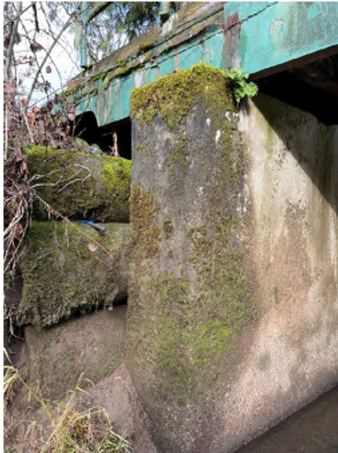
Photo 4 – Gordy Jolma No 8 Abutment and Cantilever Railcar section
