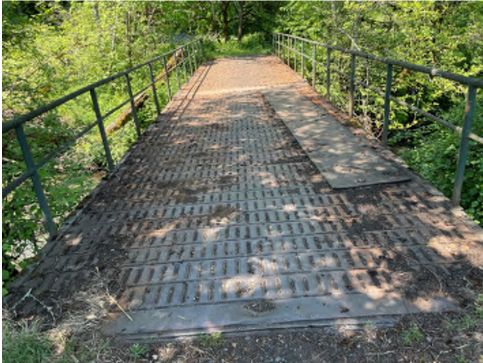
Photo 1 – Gordy Jolma No 5 Approach and Deck view.
