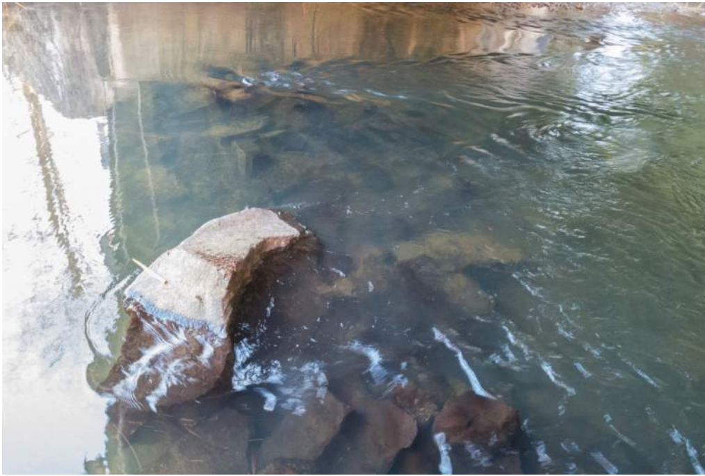
Photo 3: Smith Bridge existing riprap under bridge
