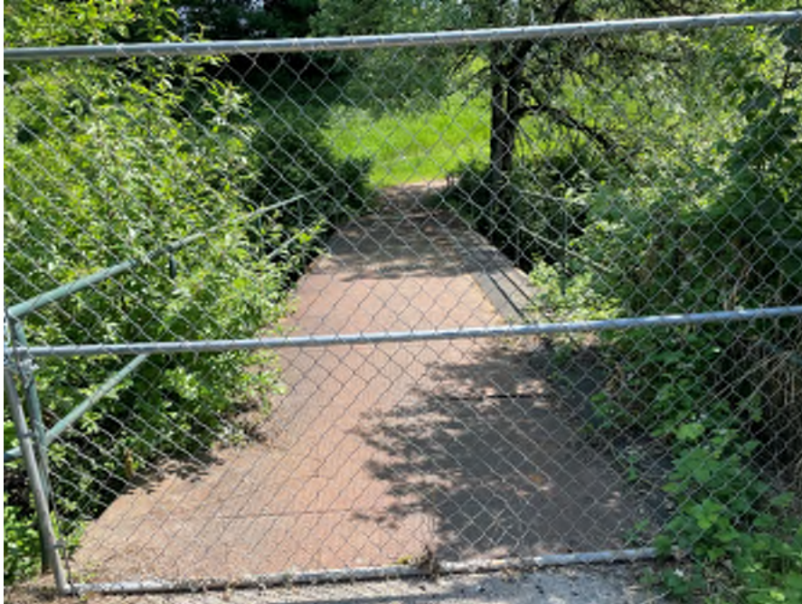
Photo 1 – Gordy Jolma No 3 Deck view.
