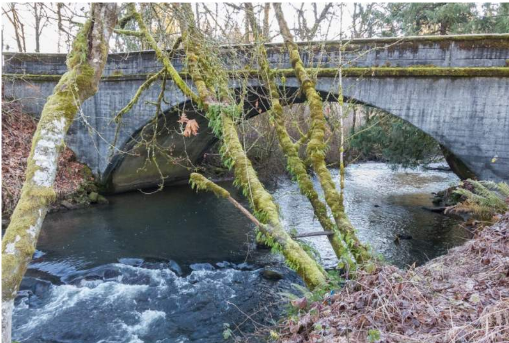
Photo 2: Salmon Creek Bridge – Looking upstream
