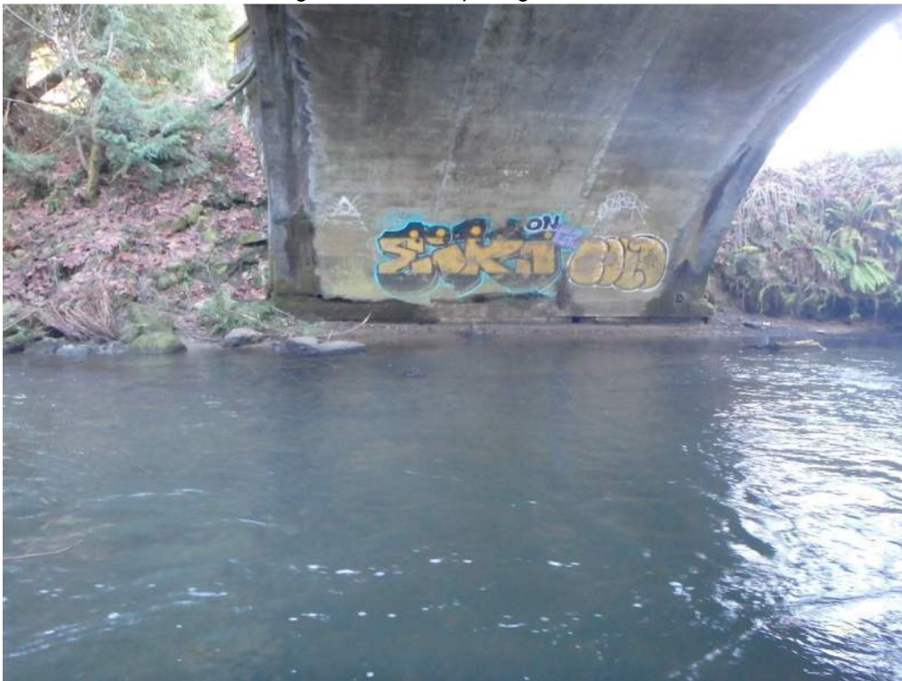
Photo 4: Salmon Creek Bridge – South Abutment
