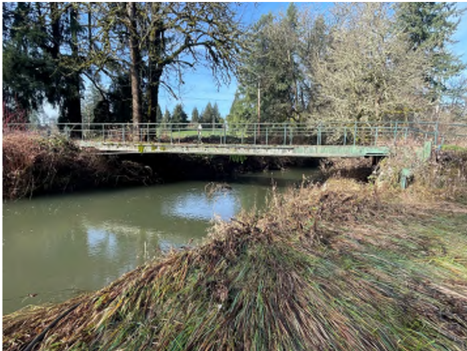
Photo 2 – Gordy Jolma No 6 Elevation view.
