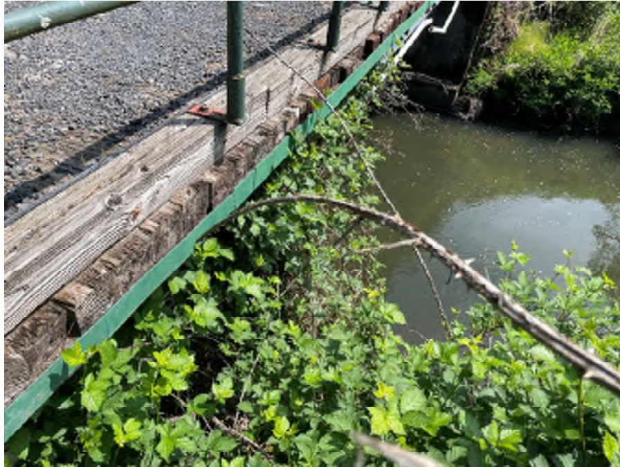
Photo 3 – Gordy Jolma No 2 Side view of deck and Abutment
