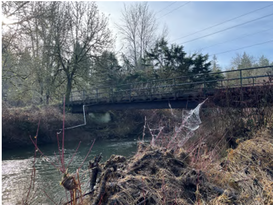
Photo 2 – Gordy Jolma No 7 Elevation view.
