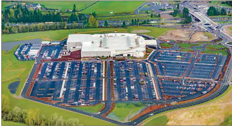
Ready to open! An aerial view of the ilani casino resort looking east taken a few days before the grand opening.
